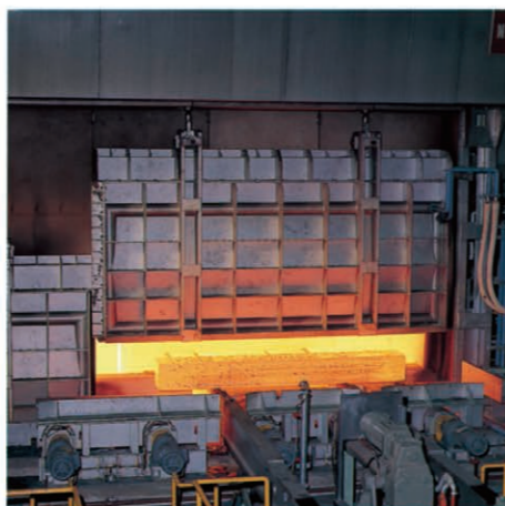
加熱設備 Heating Equipment
