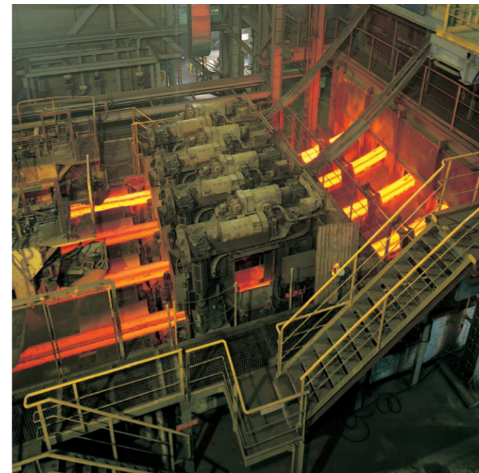
連続 casting 設備 Continuous casting equipment
