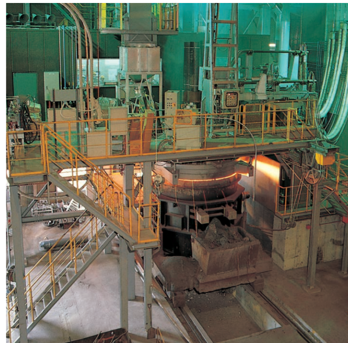
取鋼精錬 Ladle refining
