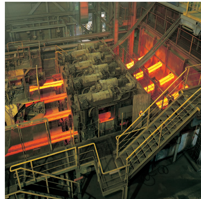
連続 casting 設備 Continuous casting equipment
